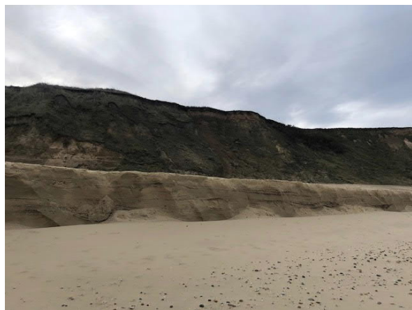
Fig 3.2D. Cliff condition and beach level at HDD.
