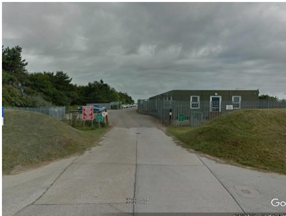
Fig 3.1C. Access from the B1159 Coastal Road.
