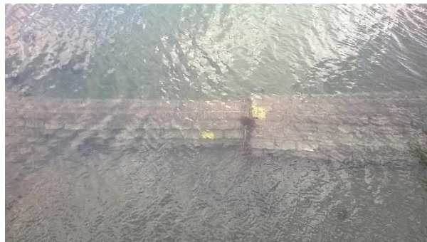
Fig 11.2D Concrete mattress being lifted from vessel. Fig 11.2E Concrete mattresses covering submerged duct.
