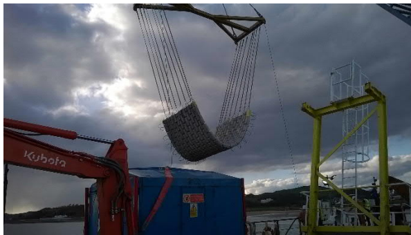
Fig 11.2D Concrete mattress being lifted from vessel. Fig 11.2E Concrete mattresses covering submerged duct.
