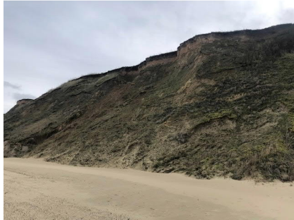
Fig 3.2F. Cliff condition at beach level.
