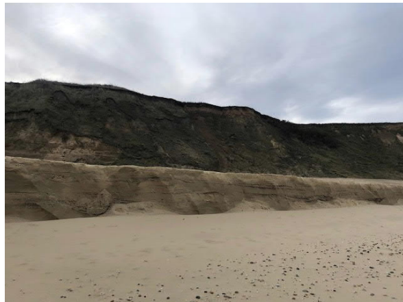
Fig 9.2C. Beach levels following sandscaping.
